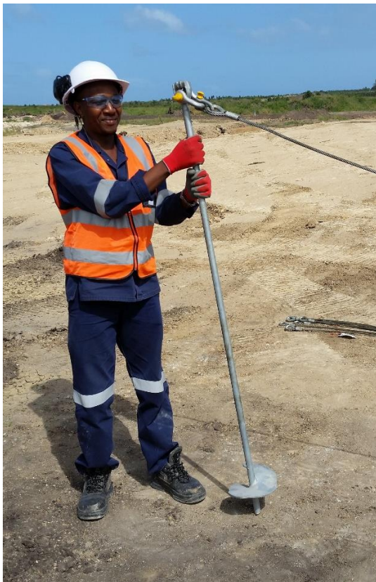
Helical anchor inserted in 2 minutes.
