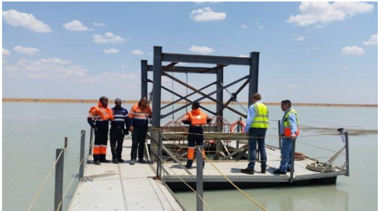
Penstock tower Walkway 6 years after installation complete (under the African Sun)
